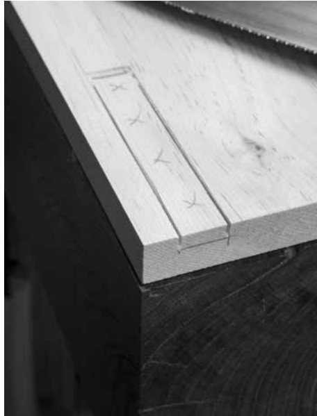
Sawn walls. If you are in a sawing mood, cut the walls with a tenon saw.
